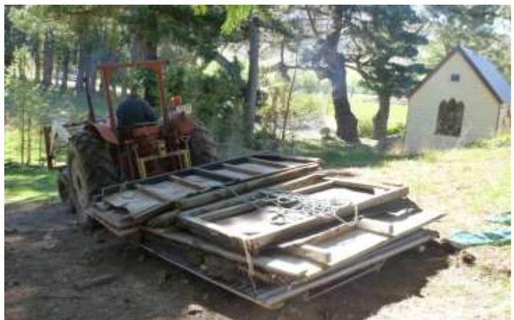
In the process of dismantling the hut it became apparent that it might have started life with a canvas roof stretched over a wooden frame as significant remnants of the canvas remained under the later addition of tarpaper and corrugated iron. Early research suggests this may be an unusual early building technique.
